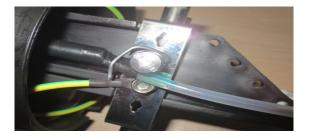
4. Remove the loose tube of the cable and clean the bare fibers. Put them through the transparent PE tube strip by strip, using PVC tape to wrap the end of the PE tube and cable.
