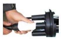
8. Clean the cable surface and ports.
